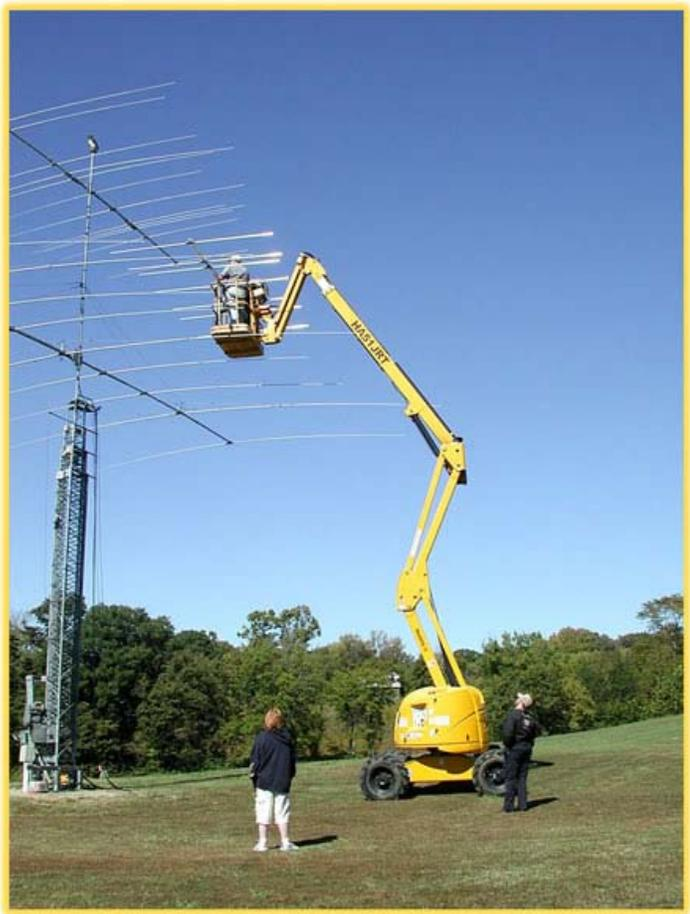
**Recent antenna raising party at the QTH of Jamie WB4YDL. A Force 12 EF-706 7-element 6 meter yagi was positioned in between two larger yagis using a self-propelled boom lift. That's Jamie riding with Glenn N4MJ in the bucket and Stan W4RB with a grandson of Glenn's observing.**
